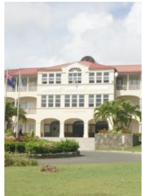
The H. L Stoutt Community College was built by the VIP Administration.
